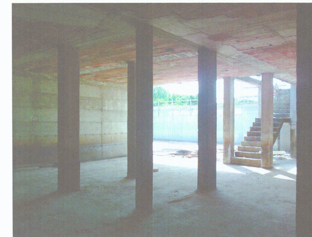
12* Interno, piano interrato
